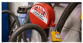
This single piece lockout device has an adjustable design that provides a secure fit when locking out T-handle ball valves on PVC pipes.
